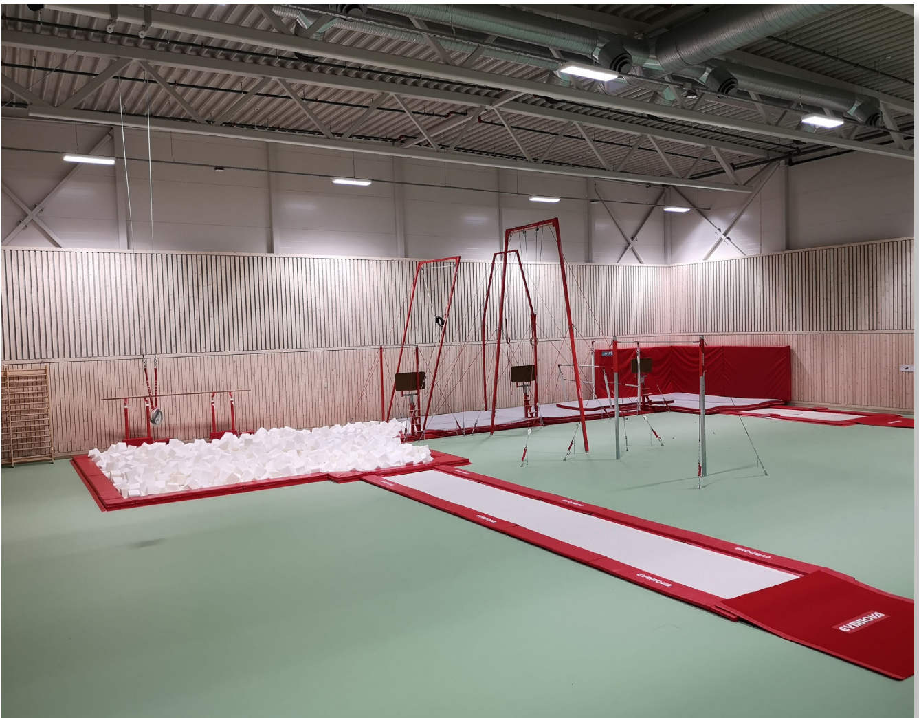
Construction of a combined pit: full built-in landing pit and sunken landing pit with foam cubes.
